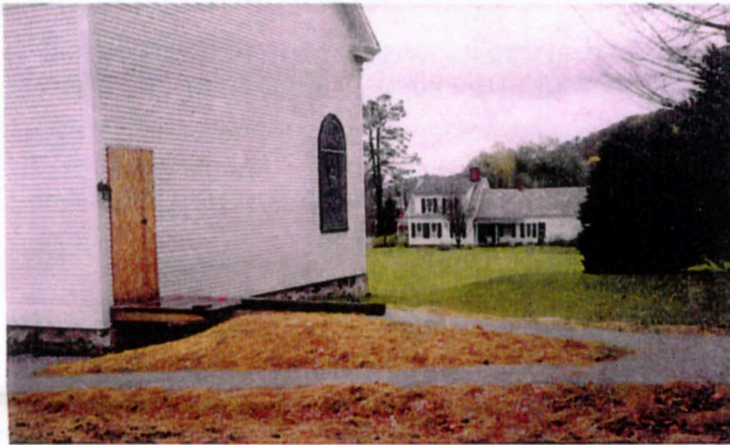
Earthen ramp under construction.
