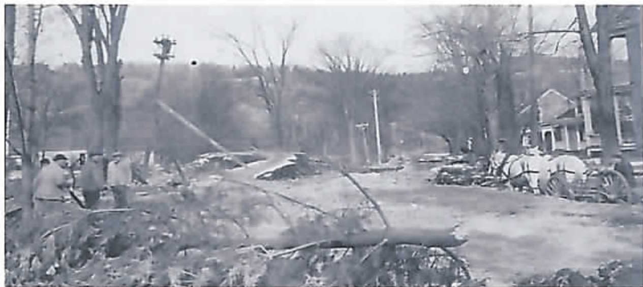
Main Street, Cuttingsville: Shown (center left) is destroyed bridge over Mill River in Cuttingsville, which is Route 103 today, looking up School Street. At left, from l-r are Merritt H. Ridlon, George Ridlon and Clayton Stewart. At right, Merritt Ridlon's team of horses with Lloyd Stapleton.
